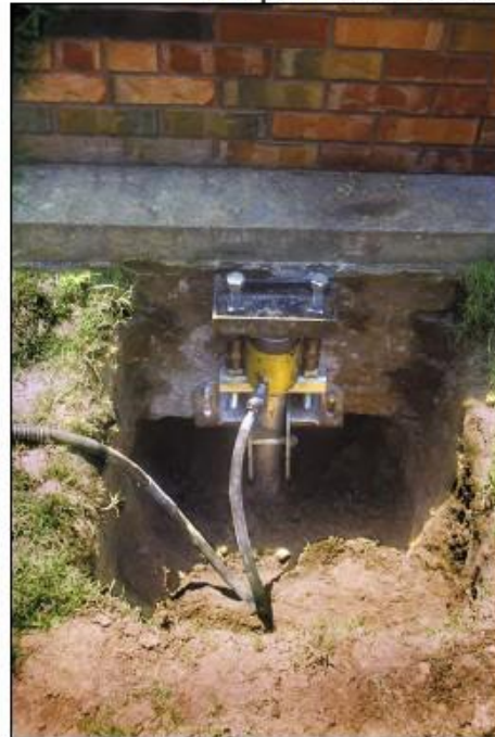
Raising Building with Repair Brackets
