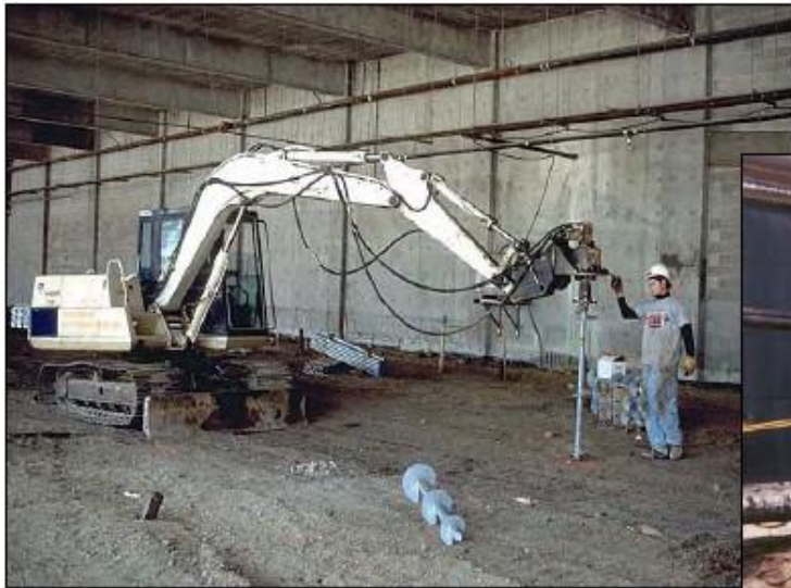
Screw Piles Supporting Structural Slab
